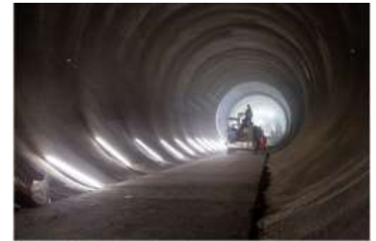
© Tollerham Court Road platform tunnels_100746
