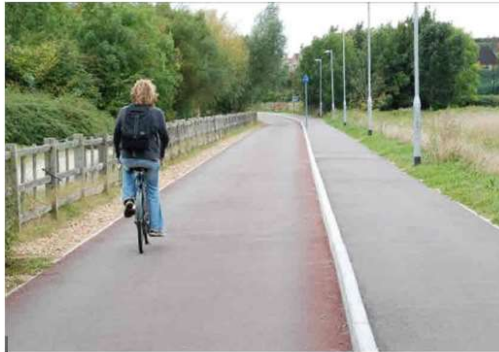
Figure 2.3.2.2 Cycle track and Footway Separated by Level with Good Quality Surface and Lighting
