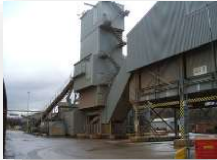
Collect from Asphalt Plant
