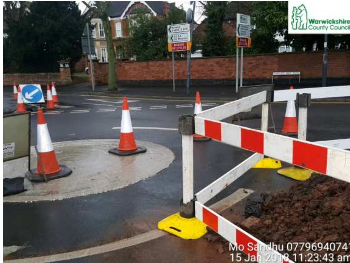
Restricted movements around the Mini Roundabout.
