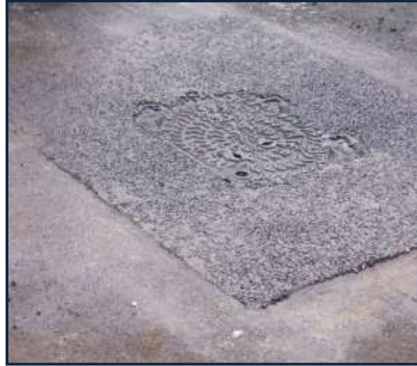
Compacted finish – May 2008
