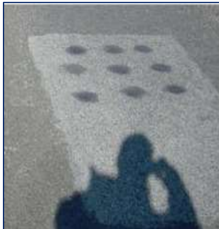
Patch in good condition Dec 2014
