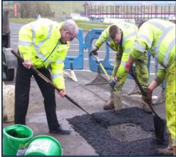
Viafix repair being made
